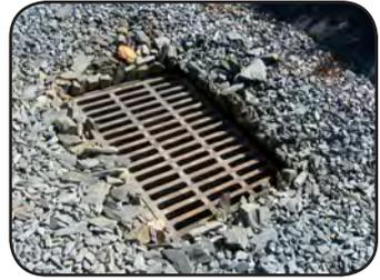
*Figure 55. Drainage tiles lead to underground pipes that carry water to the containment structure*
