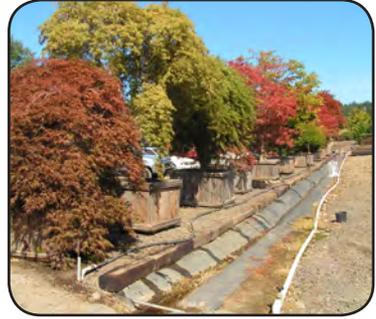
Figure 54. Conveyance ditches carry water to containment structures
