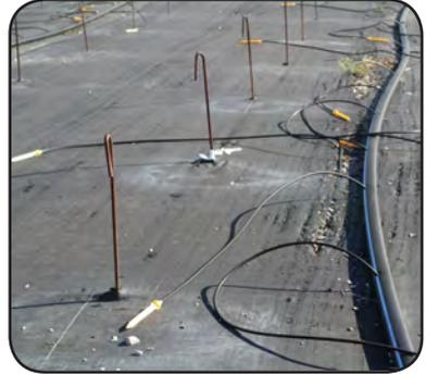
*Figure 35. If not kept out of pathways, emitters can become a tripping hazard for workers*
